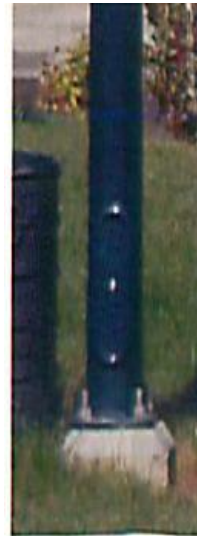
Smooth light pole base
